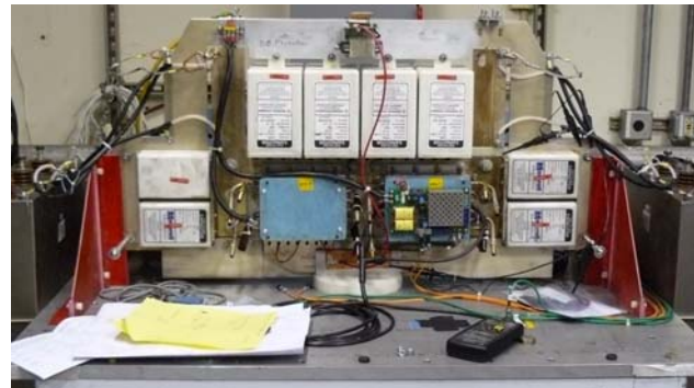
Figure 2: Existing H-bridge switch plate on SLAC test stand.
