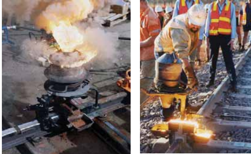
Figure 1: Thermite welding in the joining of rail tracks [1].
